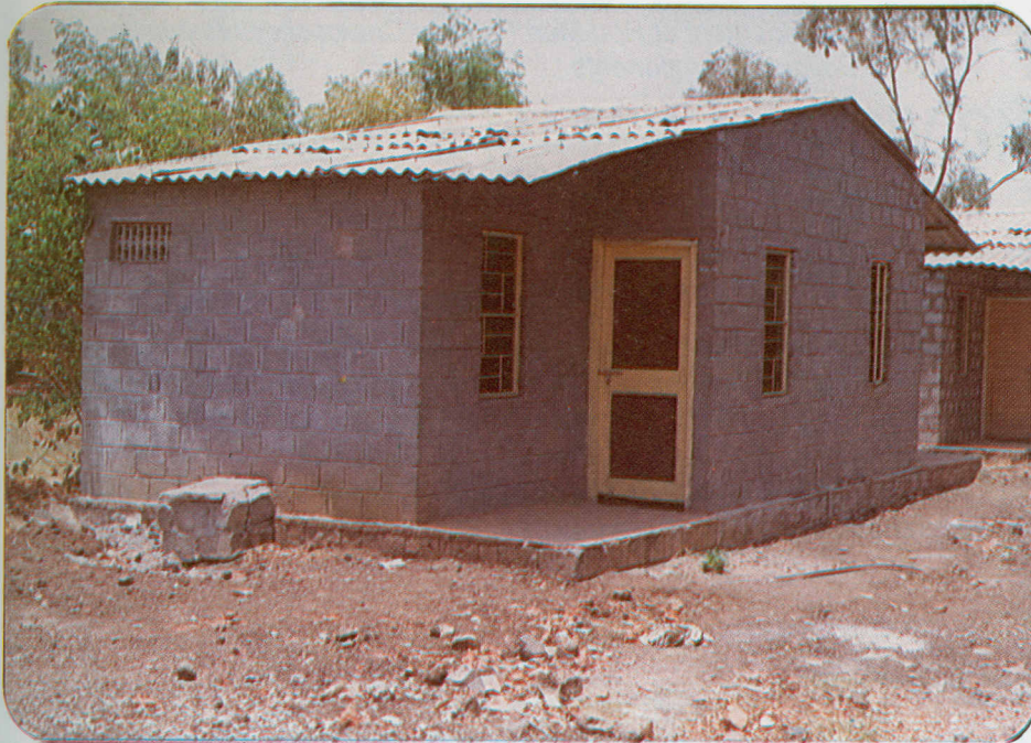
Typical Low-Cost Demonstration Housing Unit
